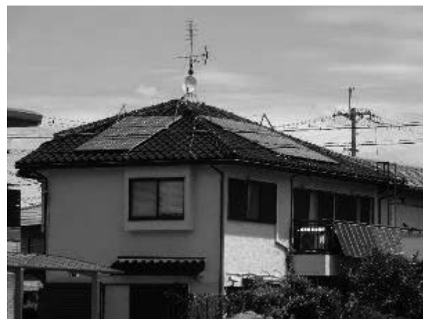
Fig. 10 The Kuwano PV Plant after 30 years of operation.
