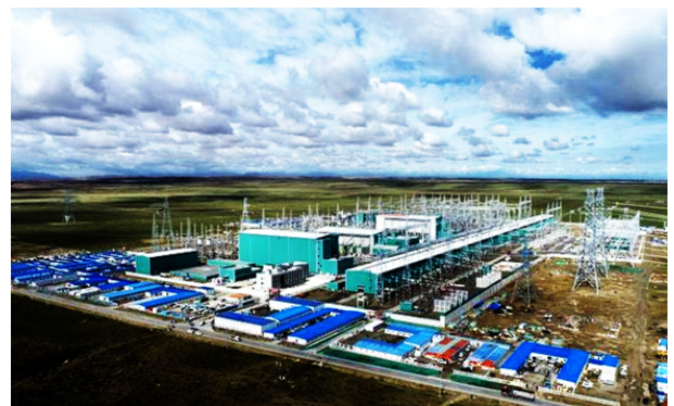
Fig.12 Aspects of Qinghai-Henan ±800 kV HVDC converter
