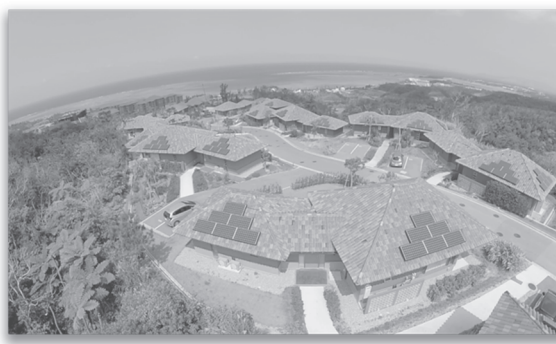
Fig. 1 A DC-based Open Energy System (DCOES) was installed on the OIST campus, Okinawa.
