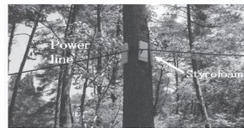
Fig. 10 Supply of electric power using a tree
