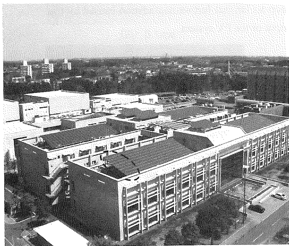
Fig.1 The PV system discussed in this paper (indicated by broken-line circle)
