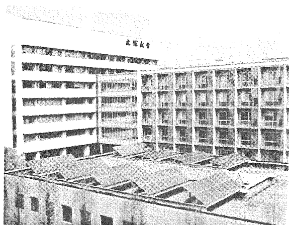
Fig.2 Exterior view of the solar arrays
