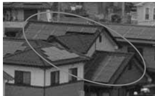
Stepped roof (large) Annual shading loss : 6.1%
